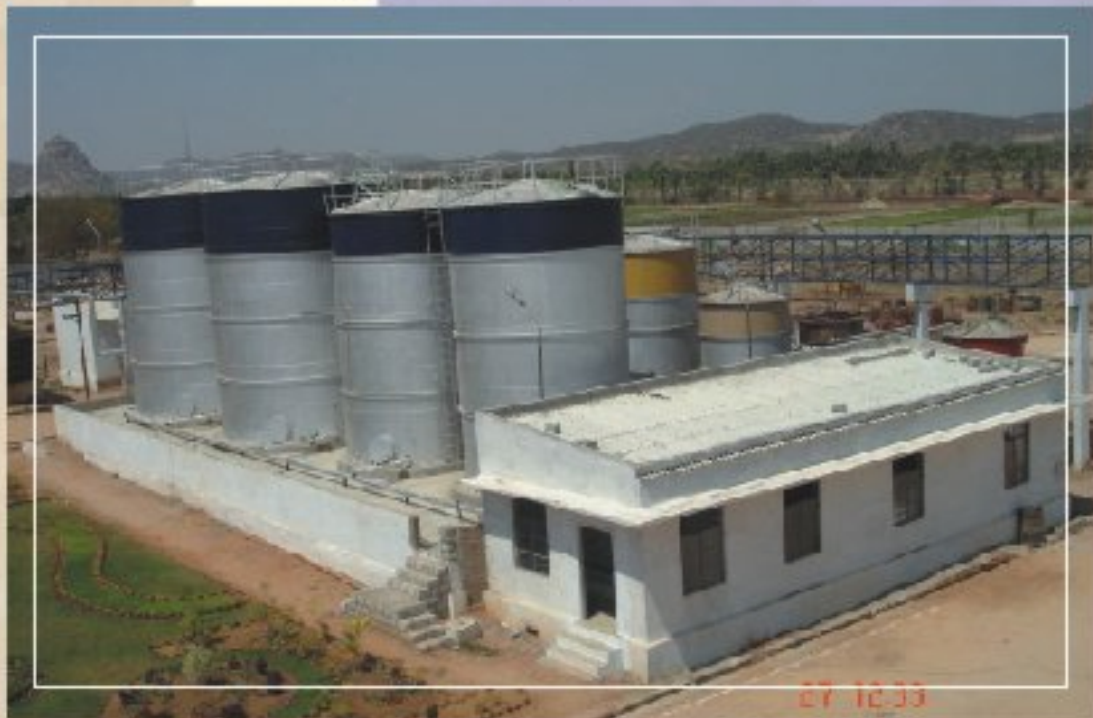
Storage Tanks at SBT Biodiesel Plant
